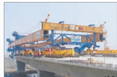
12.9 Bridge and tunnel construction
